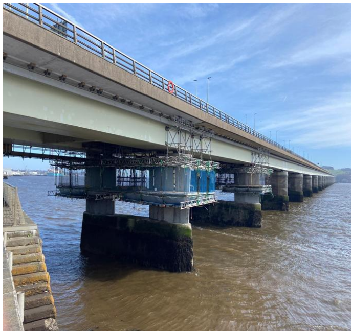
Scaffold and V-Deck Access Arrangement suspended from below bridge
